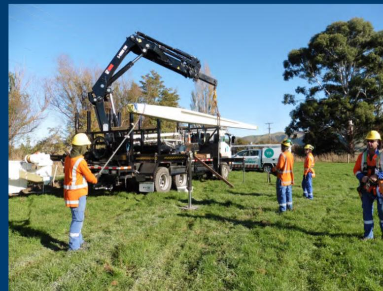
Arron testing a prototype of his insulated guidance tool.
